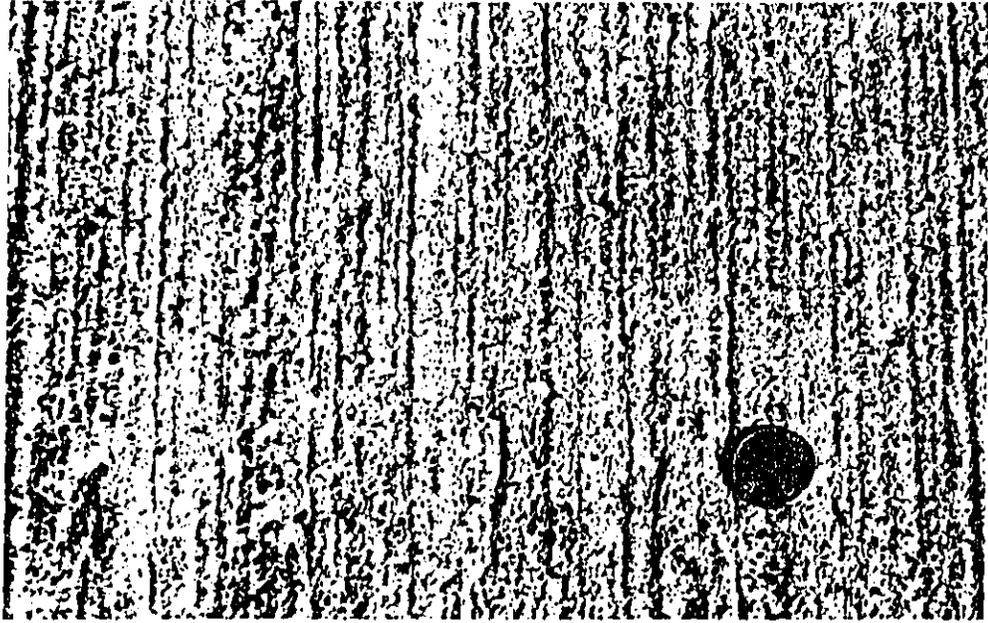
Figure 24. Rough Concrete (C3).
