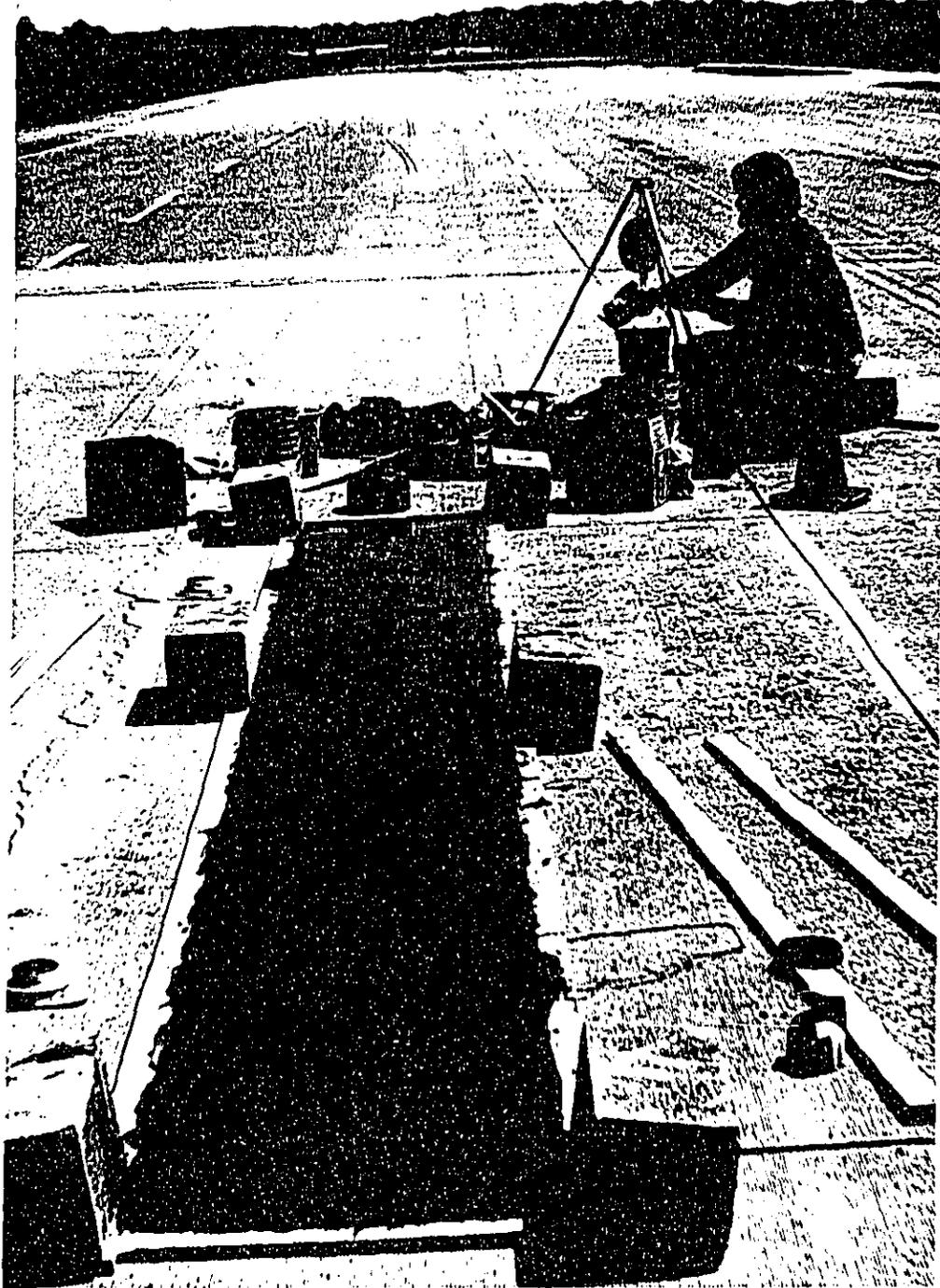
Figure 2. Making Rubber Impression of Pavement.
