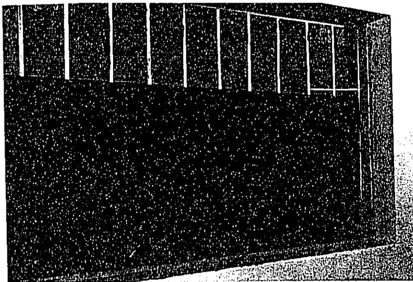
Figure 2. Application of building felt and wire mesh prior to stucco application.
