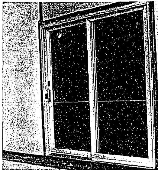
Figure 13. Plastic coated wood sliding glass door.
