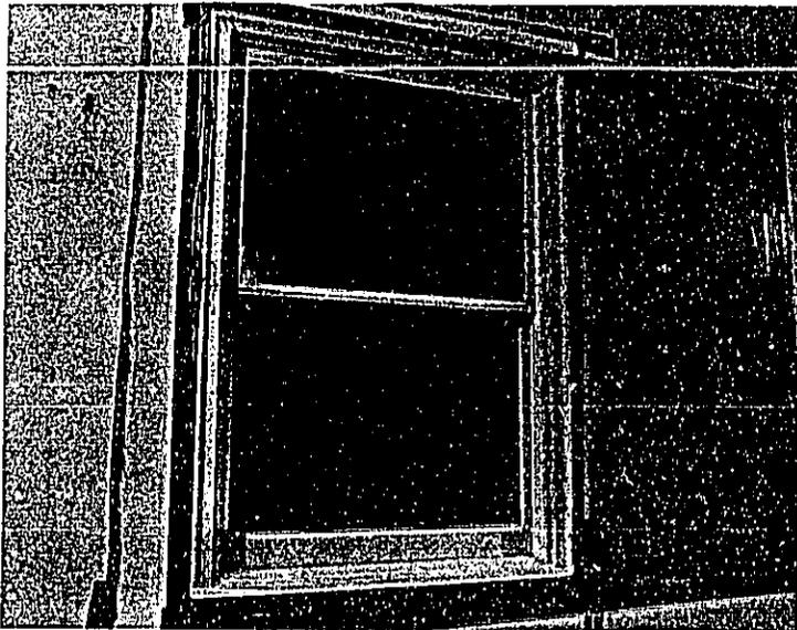
Figure 7. Wood double-hung window installed in filler wall.
