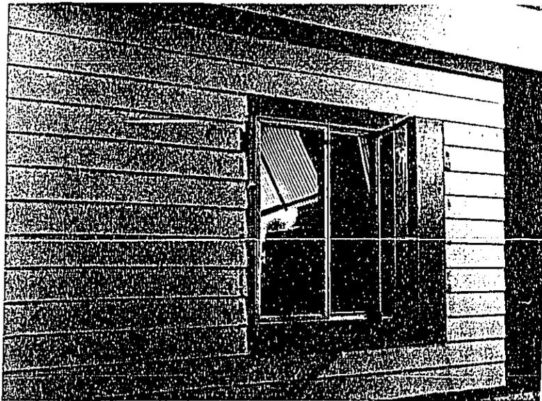
Figure 11. Plastic coated wood operable casement window.
