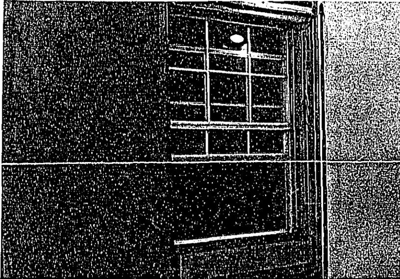
Figure 8. Aluminum single hung window.
